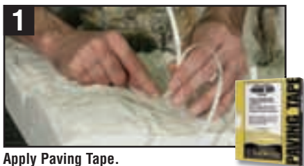
1 Apply Paving Tape.
